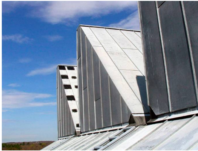
Figure 1.3 A Building with Sawtooth Roof Located in Wellesley, MA
